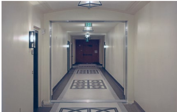
[58] Fire doors that retract into the walls have been installed here (not visible in photo) preserve the historic character of this corridor.
