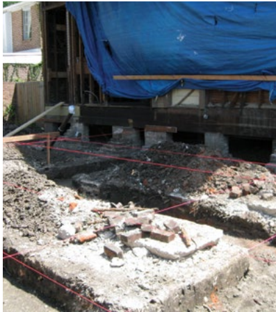
[45] Undertaking a survey to document archeological resources may be considered in some rehabilitation projects when a new exterior addition is planned.
