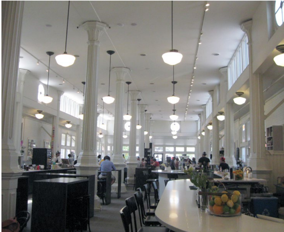
[14] Interior cast-iron columns have been cleaned and repainted as part of the rehabilitation of this historic market building for continuing use.
