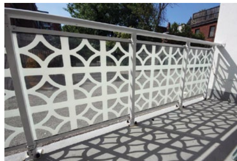
[59] (a-b) The decorative concrete balcony railings on this 1960s building did not meet life-safety code requirements. They were replaced with new glass railings with a fritted glass pattern matching the original design—a creative solution that satisfies codes, while preserving the historic appearance of the building when viewed from the street (c-d). Photos: (a, b, d) ERA Architects, Inc.; (c) Nathan Cyprys, photographer.
