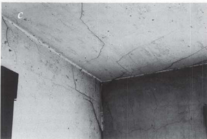
Fig. 7 (a) to (d). A series of photographs taken in different rooms of an early 20th century house in West Virginia reveal a variety of plaster wall surface problems, most of which can easily be remedied through sensitive repair: Hairline cracks (a) in an otherwise sound wall can be filled with joint compound or patching plaster. The wall can also be canvassed or wallpapered. Stress cracks (b) in plaster over a kitchen door frame can be repaired using fiberglass mesh tape and joint compound. Settlement cracks (c) in a bedroom can be similarly repaired. The dark crack at the juncture between walls, however, may be a structural crack and should be investigated for its underlying cause. Moisture damage (d) from leaking plumbing on the second floor has damaged both wallpaper and plaster in the dining room. After fixing the leaking pipes, the wall covering and rotted plaster will need to be replaced and any holes repaired. Photos: Kay Weeks.
