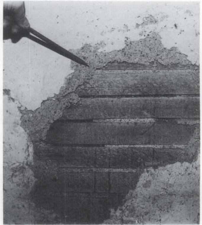
Fig. 8. Too much aggregate (sand) and not enough cementing material (lime or gypsum) in the base coat has made this plaster surface weak and crumbly. Besides losing its key with the lath, the layers are disintegrating. It will most likely need to be totally removed and replaced with all new plaster. Photo: Marylee MacDonald.
