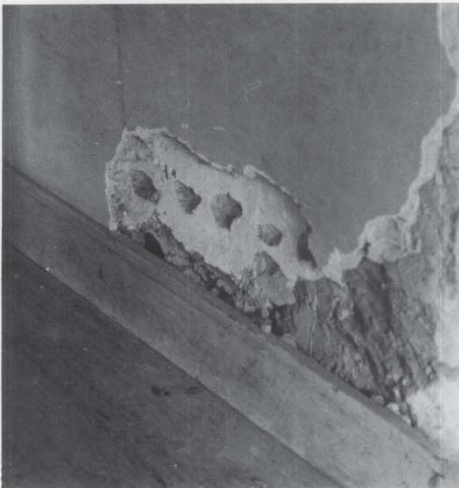
Fig. 4. The builders of this mid-18th century house installed the baseboard moulding first, then applied a mud and horse hair plaster (called paling ) to the masonry wall. Lime was used for the finish plaster. Also shown are the hacking marks which prepared the wall for a subsequent layer of plaster. Photo: Kay Weeks.
