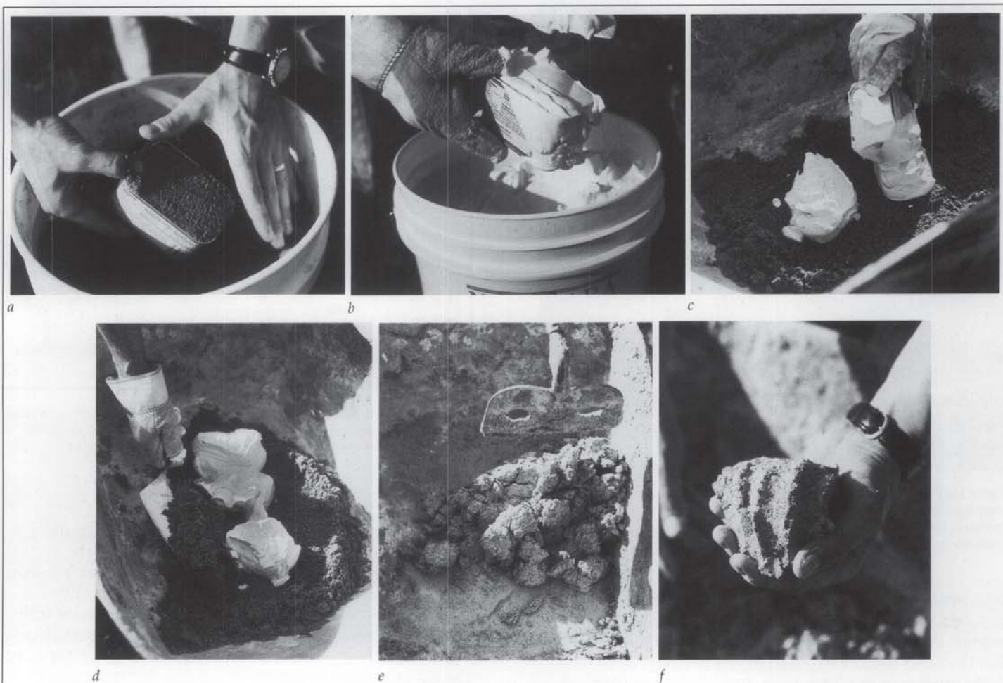
Figure 14. Mixing mortar using lime putty: (a) proportioning sand; (b) proportioning lime putty; (c) placing lime putty on top of sand; (d) mixing sand over lime putty; (e) hand mixing mortar; and, (f) sample of mortar after mixing. Photos: John P. Speweik.
