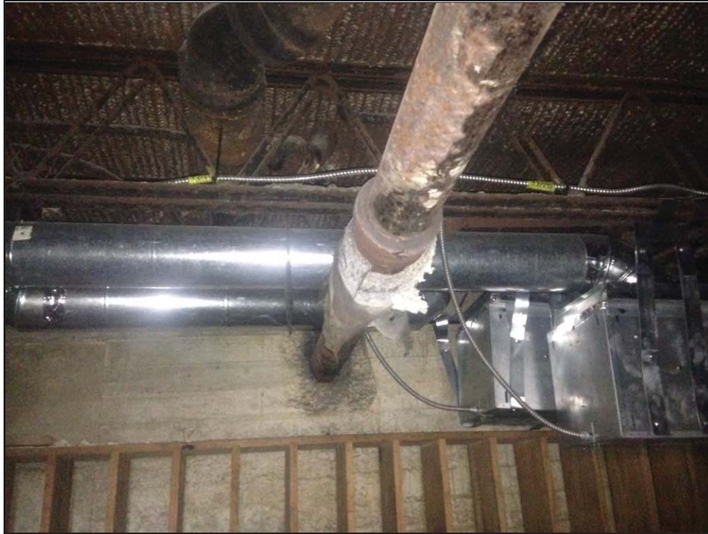
Photo 3: New ductwork, pipe run with asbestos-containing insulation (moist to the touch), and wood shelving (elevated moisture content) located in the basement. The insulation and wood shelving should be removed from the basement to prevent future mold growth.
