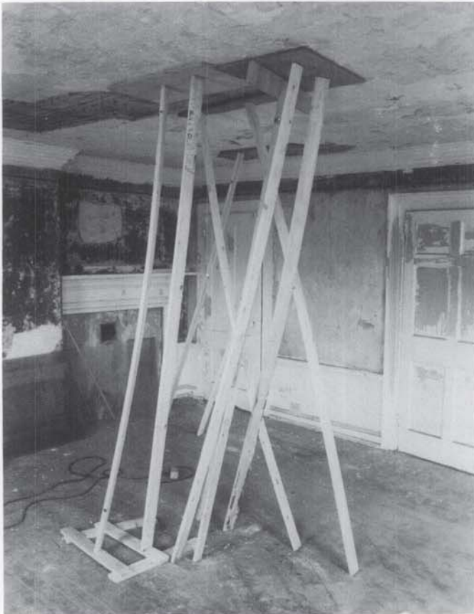
Fig. 15. When ceiling repairs are made with wet plaster or with an injected adhesive mixture, the old loose plaster must be supported with a plywood brace until re-keying is complete. Photo: John Leeke.
