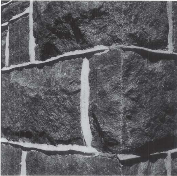
Figure 15. The profile of the repointed joints on the left replicate the historic joints around the corner to the right on the front of this stone building in Leesburg, VA. The contractor's pride in the repointing work is evident by the signature in the vertical joint. Photo: Anne Grimmer.
