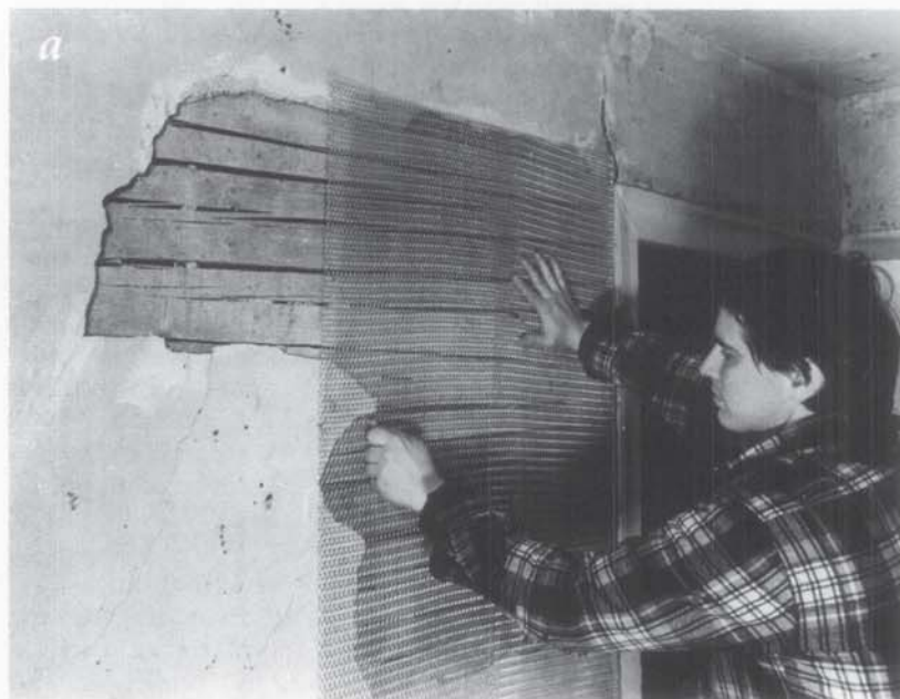
Fig. 10 (a) and (b). In this New Hampshire residence dating from the 1790s, the original plaster was a single coat of lime, sand, and horsehair applied over split lath. A one-coat repair, in this case, is appropriate. To the left: a flat sheet of galvanized expanded metal lath is placed over the patch area and an outline marked with a large soft lumber crayon. The metal lath is then cut to fit the hole and nailed to the lath. To the right: the edges of the original plaster and wood lath beneath have been thoroughly soaked with water. A steel trowel is used to apply the plaster in large, rough strokes. Finally, it will be scraped and smoothed off. Because only one coat of plaster is used, without a finish coat, a clean butt-joint is made with the original plaster. Photos: John Leeke.
