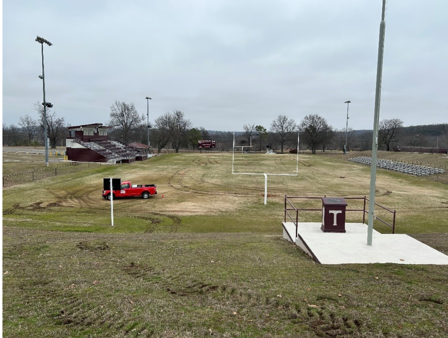
Figure 2: Northwest of the project site, looking southeast across the football field
