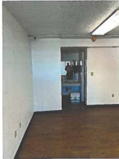
Concrete Wall Texture - Throughout 2nd Floor North
