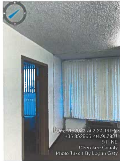
Concrete Ceiling Texture - Throughout 1st Floor North
