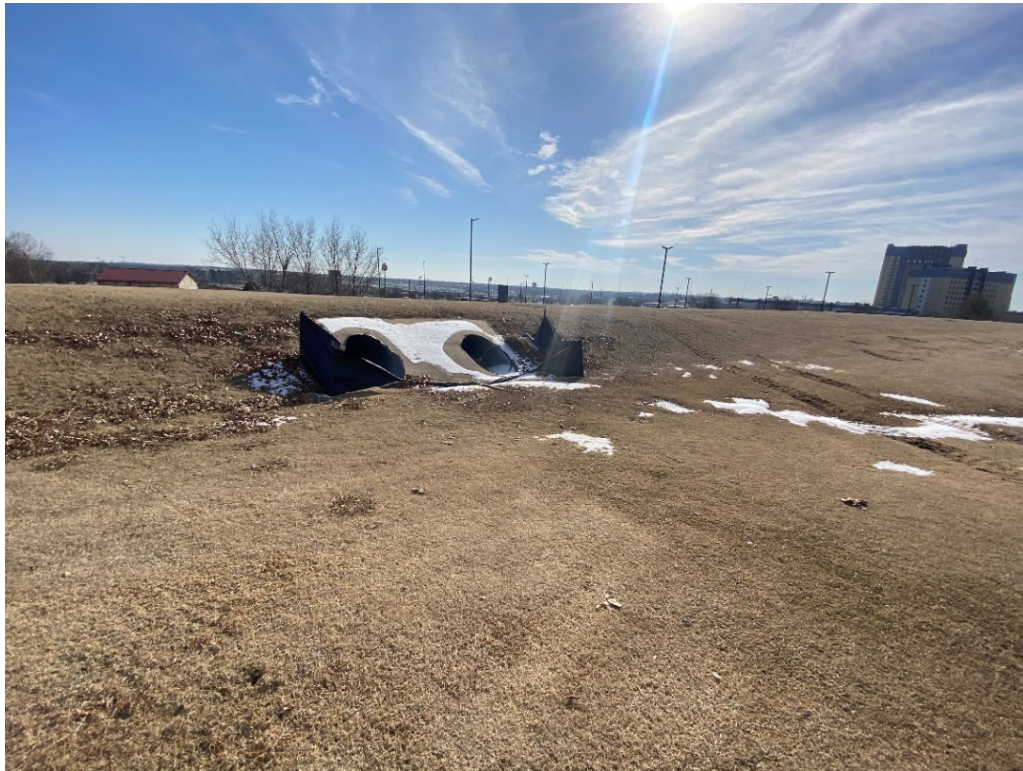
Figure 6: Underground drainage feature noted near boring P-02
