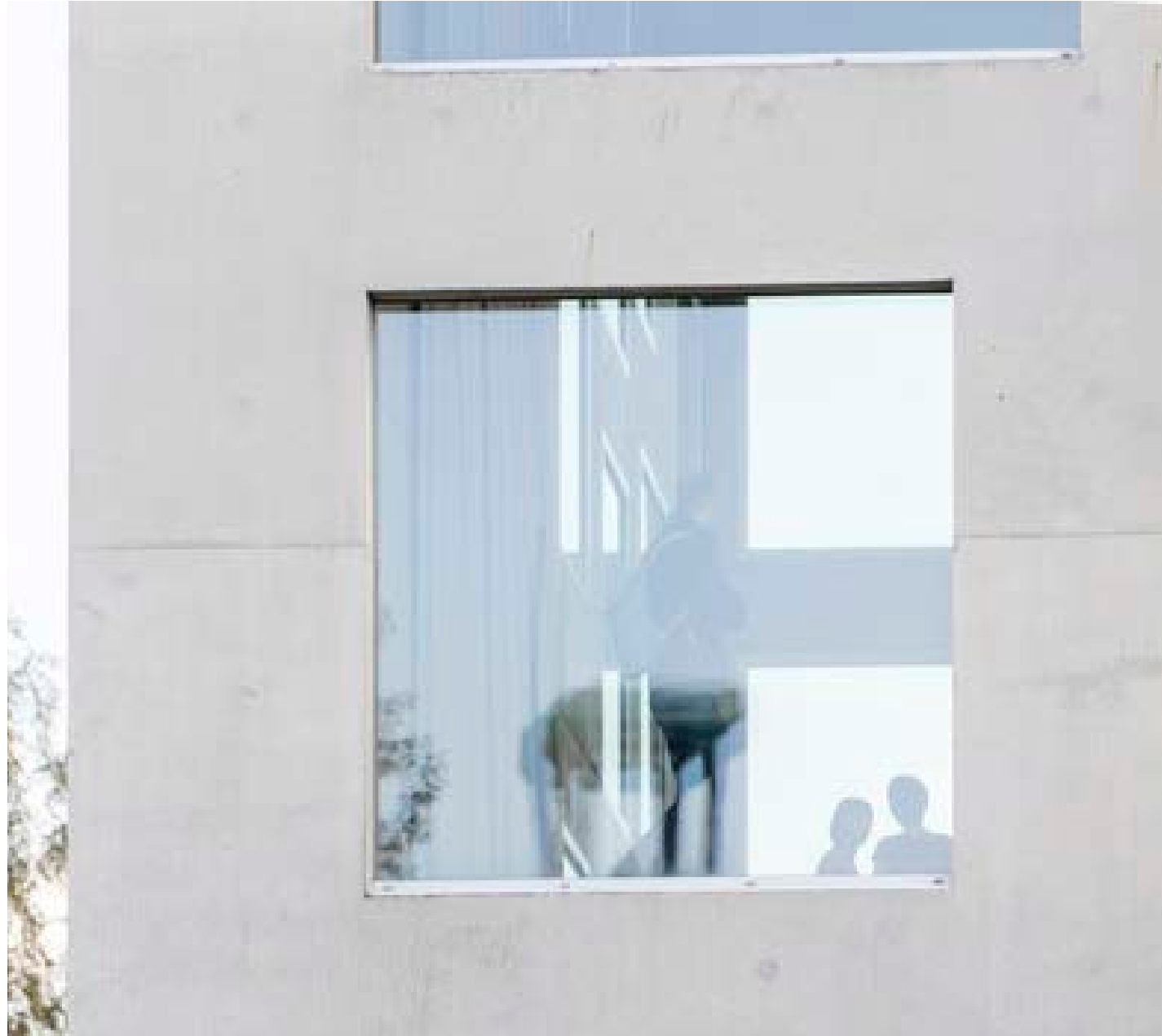
EXAMPLE OF PICTURE WINDOW IN ARCHITECTURAL CONCRETE WALL WITH MINIMAL/FLUSH FRAME EXPRESSION
