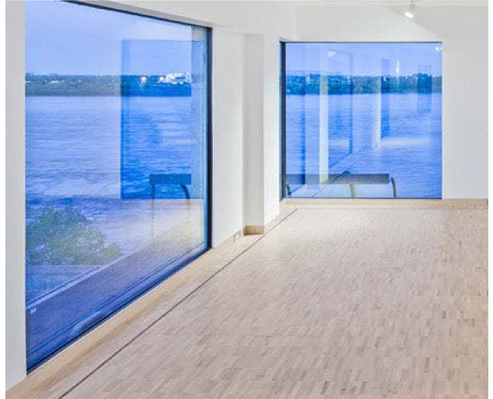
EXAMPLE OF PICTURE WINDOW IN ARCHITECTURAL CONCRETE WALL WITH DRYWALL INTERIOR CONDITION AND FOOTER FLUSH WITH FINISH FLOOR
