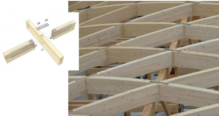
Figure 6-7 - Cafe Roof - Precedent Lamella Connection
