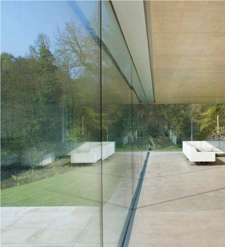
EXAMPLES OF MULLION-FREE GLAZING WITH SSG JOINTS. GLAZING ALONG BIRCH CREEK GALLERY TO BE SEGMENTED/FACETED INTO STRAIGHT SEGMENTS ALONG ARC.
