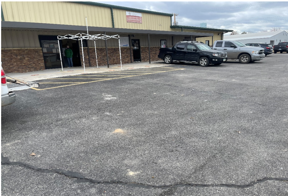
Figure 4: West side of existing facility, looking Southeast
