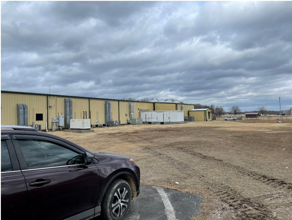
Figure 3: East side of existing facility, looking northwest at proposed cooler/freezer area
