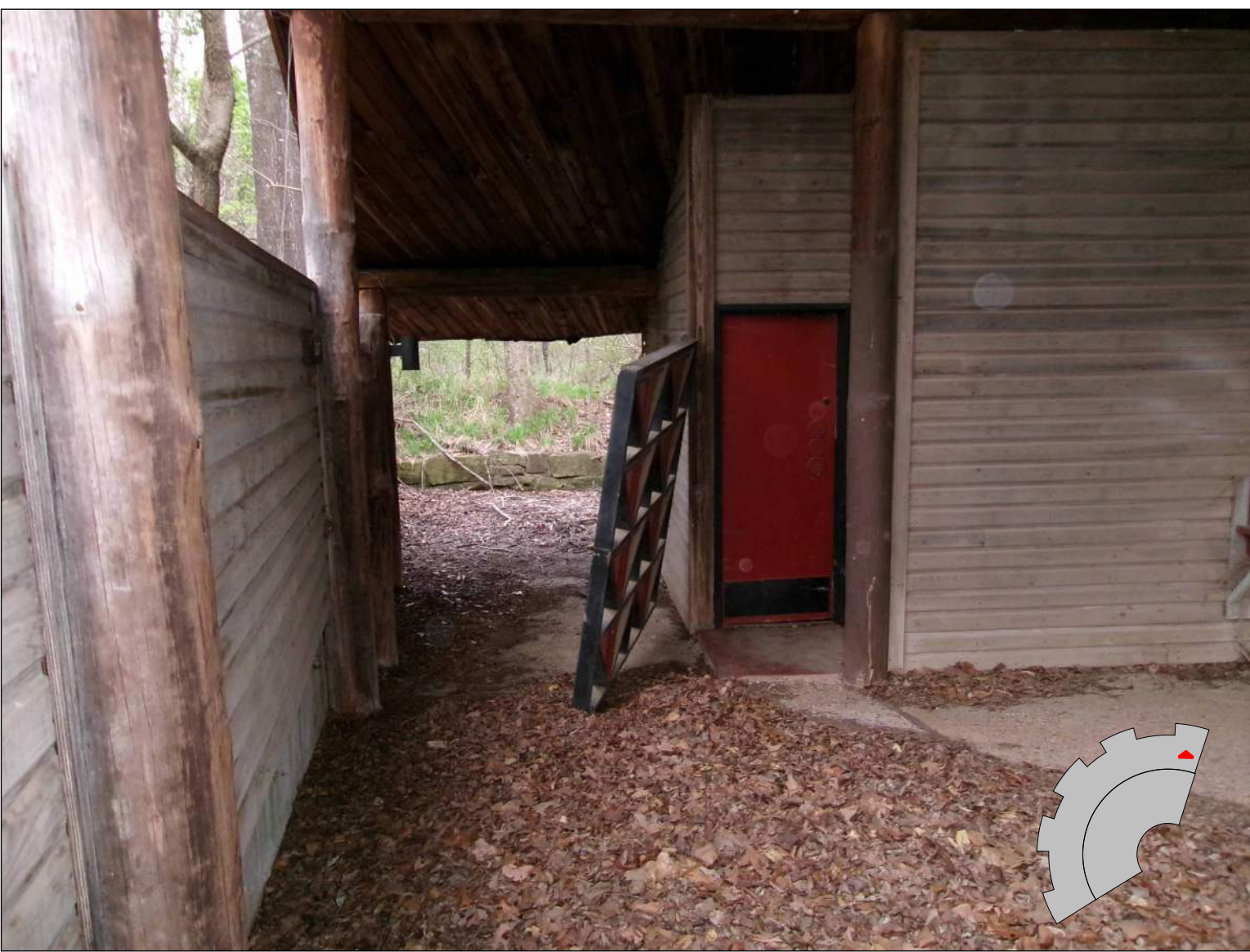
AMPHITHEATER - ROOF AND ENCLOSED AREA THERE ARE TWO INSTANCES OF THE DECORATIVE WOOD GATES SHOWN ABOVE. THESE ARE TO BE SALVAGED.
