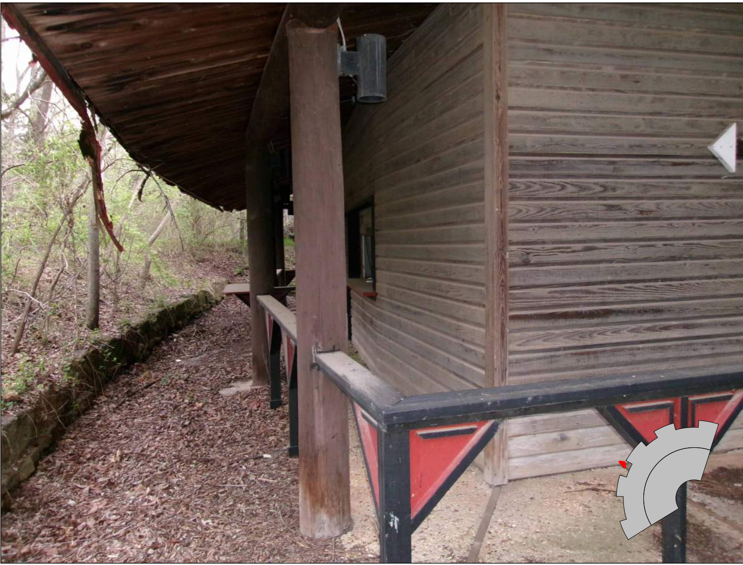
AMPHITHEATER - ROOF, STRUCTURE, AND ENCLOSED AREA REMOVE AND SALVAGE POSTS 2 AFF
