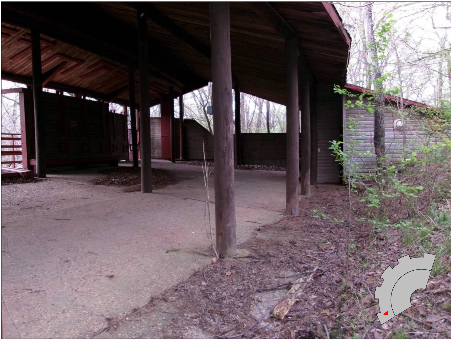
AMPHITHEATER - ROOF, STRUCTURE, AND ENCLOSED AREA REMOVE AND SALVAGE POST 2 AFF
