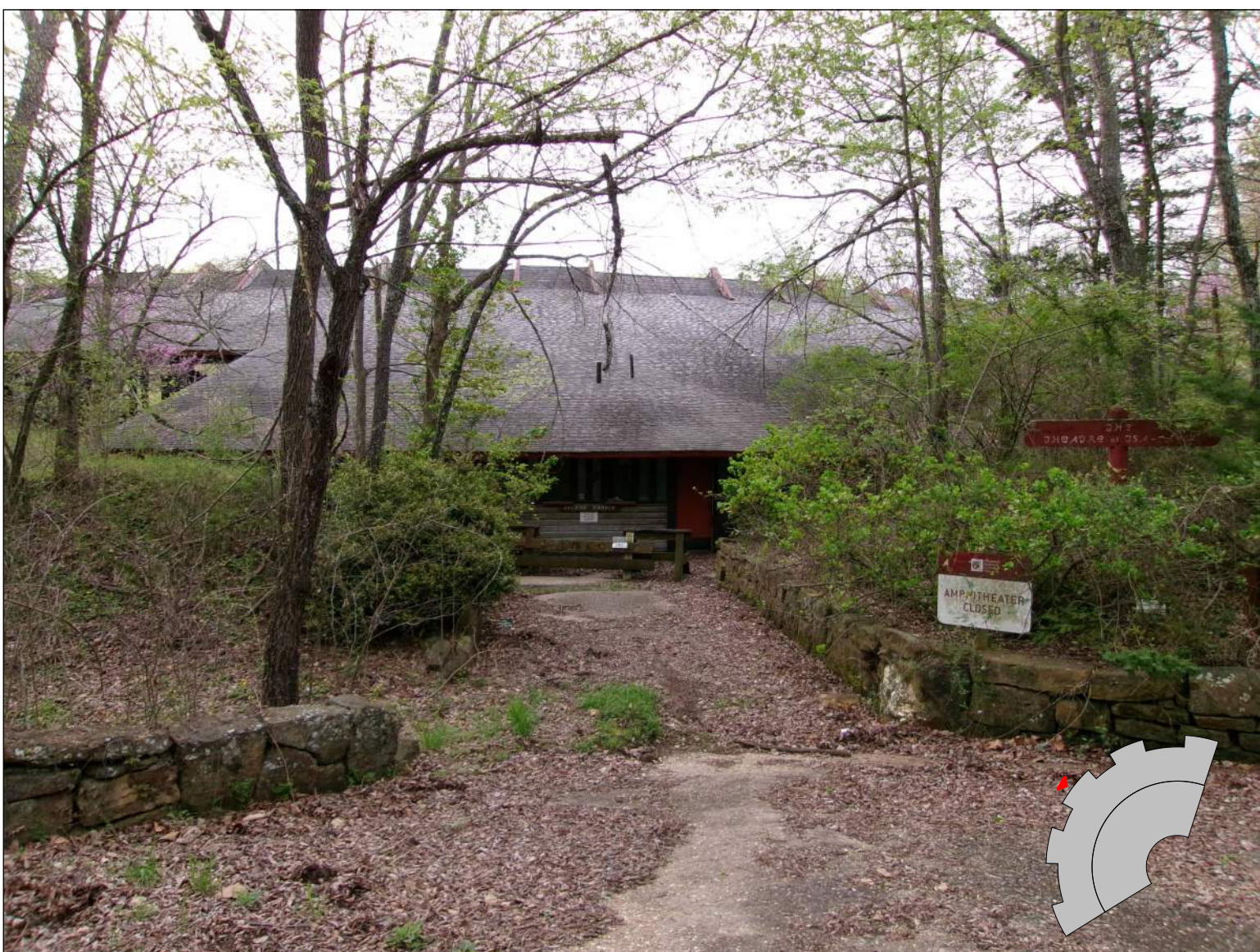
AMPHITHEATER - ENTRY AND ROOF STRUCTURE
