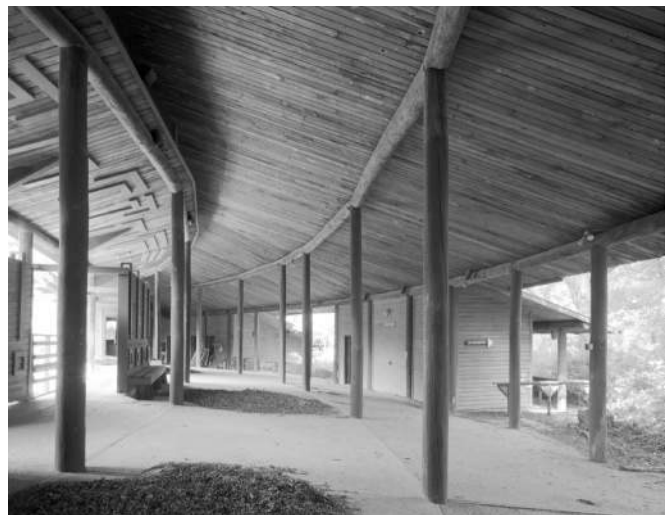
Figure 2 Log Posts and Red-Painted Wood Planks
