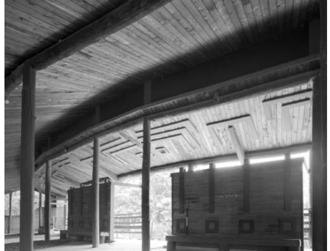
Figure 3 Log Posts and Red-Painted Wood Planks
