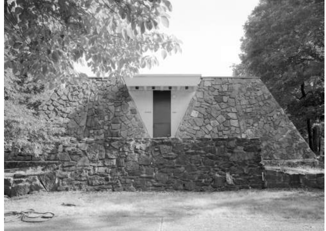
Figure 7 Sandstone Exterior Wall Panels
