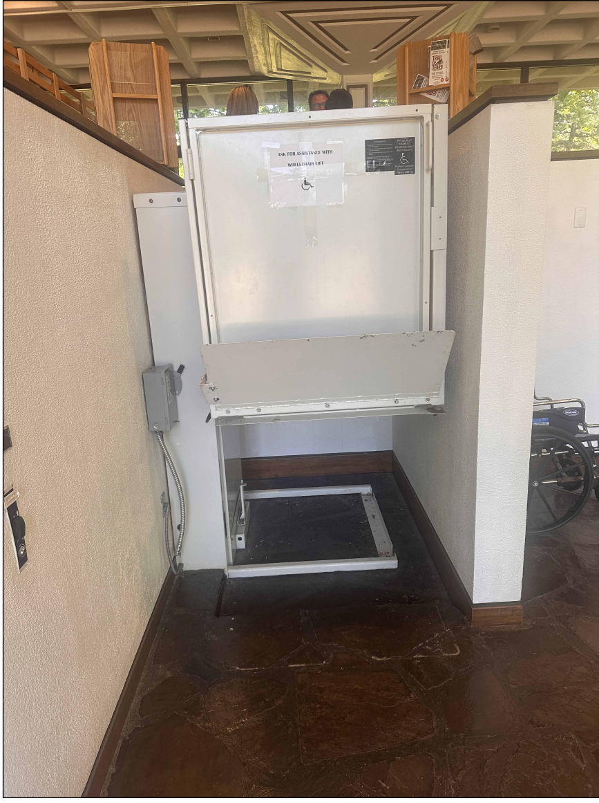
CHEROKEE NATIONAL MUSEUM - SALVAGE EXISTING CHAIR LIFT FOR OWNER TO REUSE.
