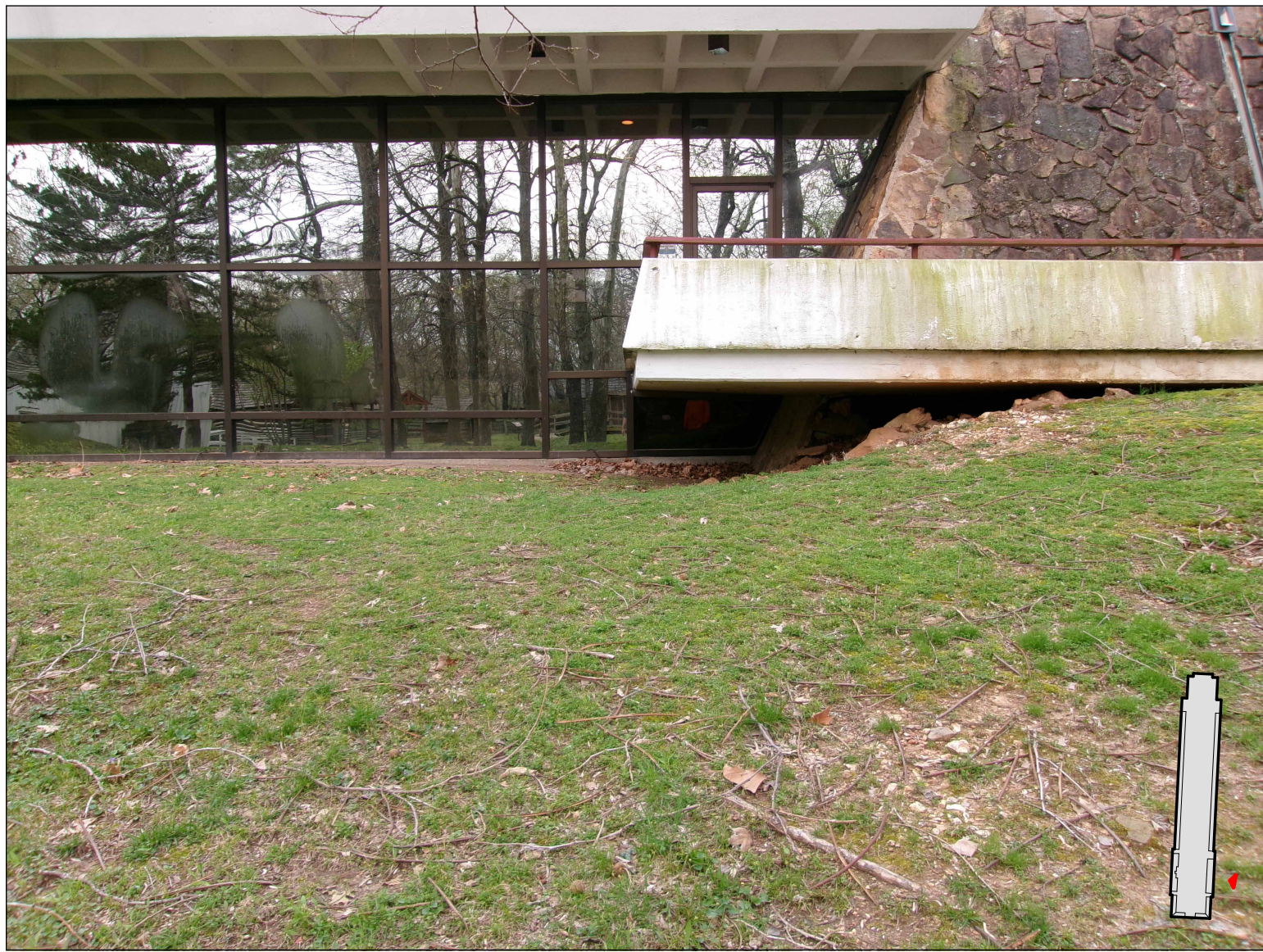
CHEROKEE NATIONAL MUSEUM - SLOPED CONCRETE WALLS WITH ADHERED STONE. STOREFRONT
