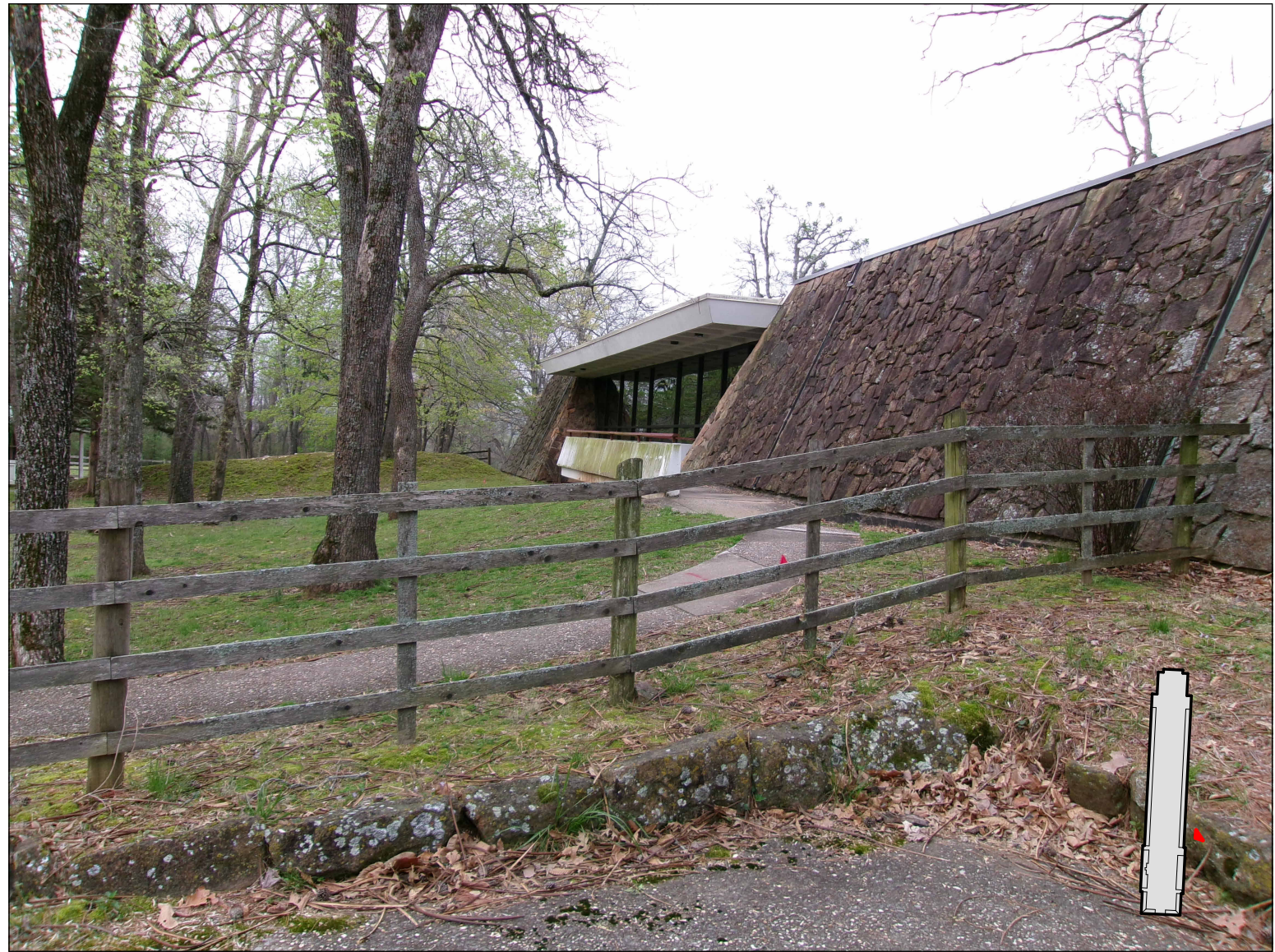
CHEROKEE NATIONAL MUSEUM - SLOPED CONCRETE WALLS WITH ADHERED STONE. STOREFRONT UNIT PRICE TO BE PROVIDED TO SALVAGE INDIVIDUAL CAST IN PLACE CONCRETE WALL PANELS AND REMOVE NATIVE SANDSTONE.
