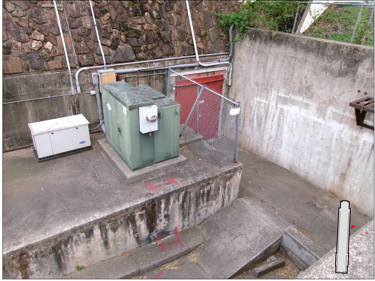
CHEROKEE NATIONAL MUSEUM - CONCRETE MECHANICAL VAULT DEMOLISH MECHANICAL VAULT AND EQUIPMENT.
