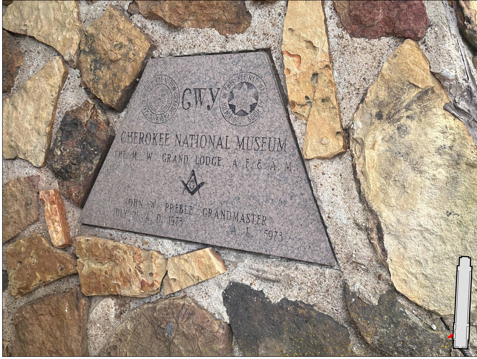
CHEROKEE NATIONAL MUSEUM - CORNER STONE TO BE SALVAGED. COPPER BOX LOCATED BEHIND CORNER STONE TO BE SALVAGED.
