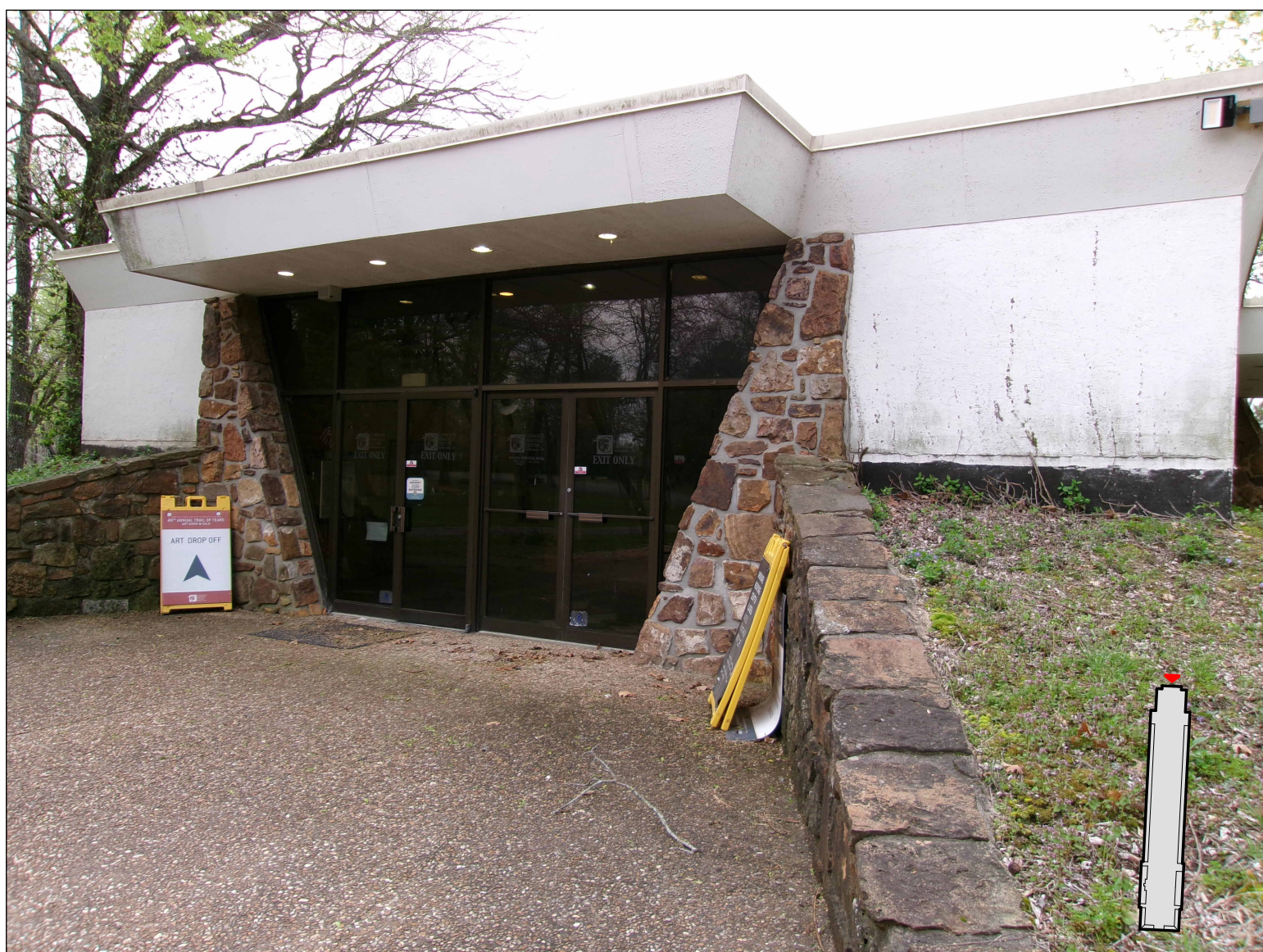
CHEROKEE NATIONAL MUSEUM - SLOPED CONCRETE WALLS WITH ADHERED STONE. STOREFRONT SALVAGE LANDSCAPING STONES FROM RETAINING WALLS.
