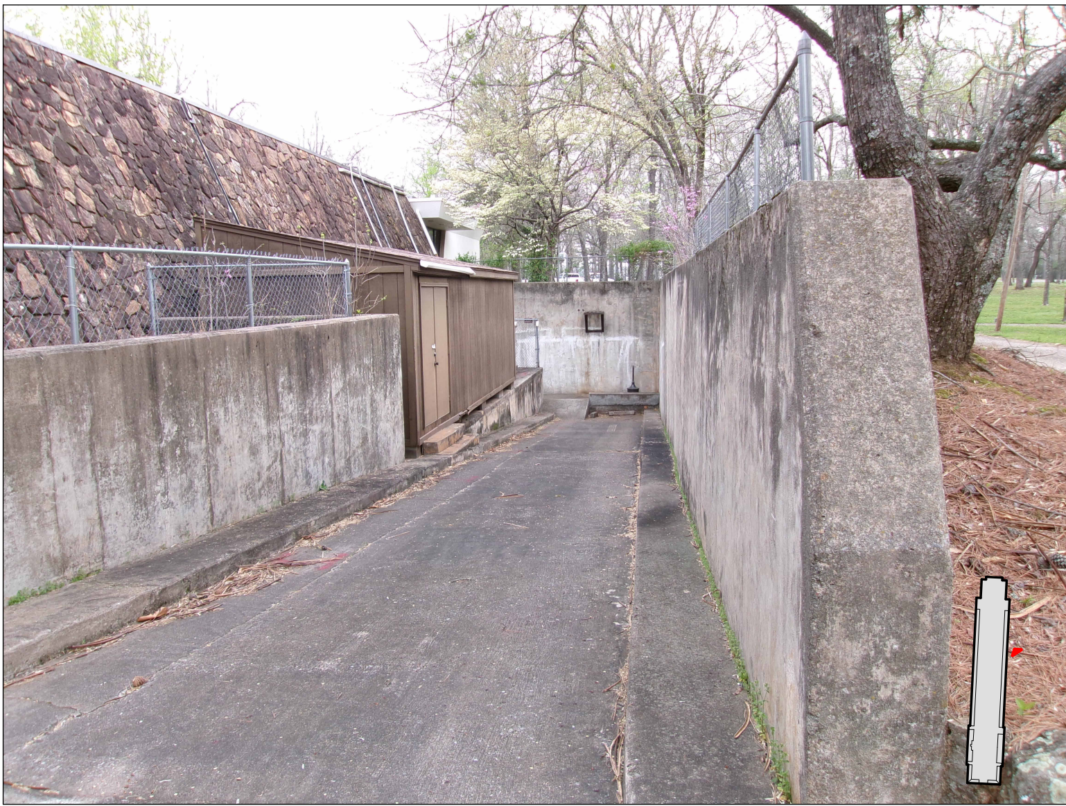
CHEROKEE NATIONAL MUSEUM - CONCRETE MECHANICAL VAULT DEMOLISH VAULT AND RETAINING WALLS
