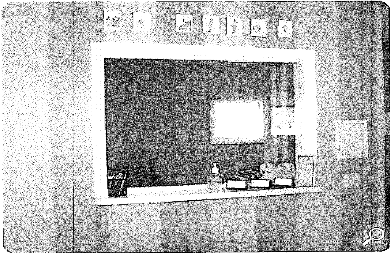
This is an example of a receptionist window with trim, shelf and dual sliding glass.
