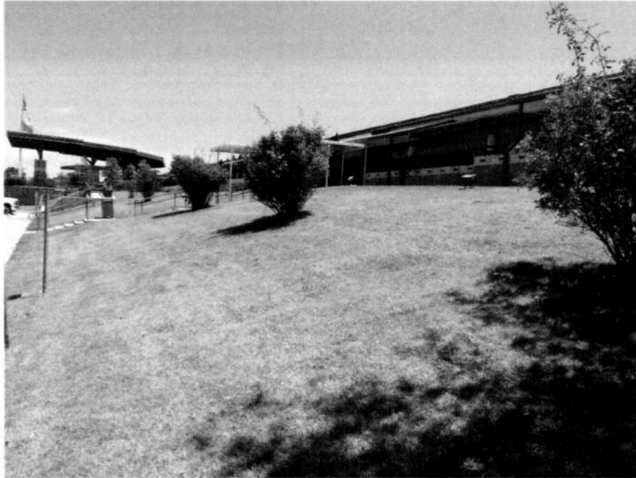
Figure 2: Photo looking east, north of the building (image dated 7/25/18)
