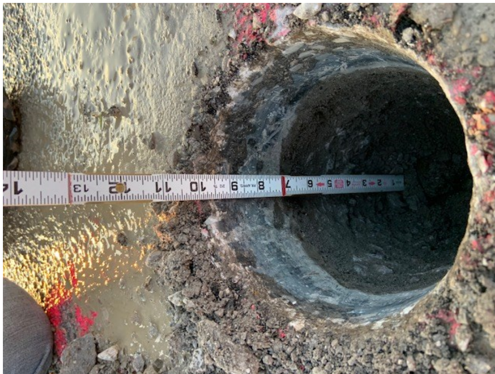
Fig. 10 – C-4: Approximately 7” of Agg Base Below Asphalt.
