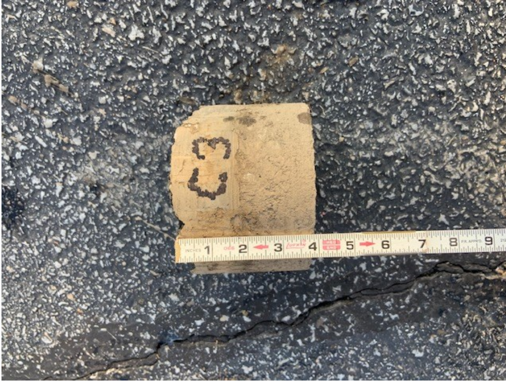
Fig. 7 – C-3: 4" Core with ~1" Left in Hole. (~5" Asphalt Thickness)
