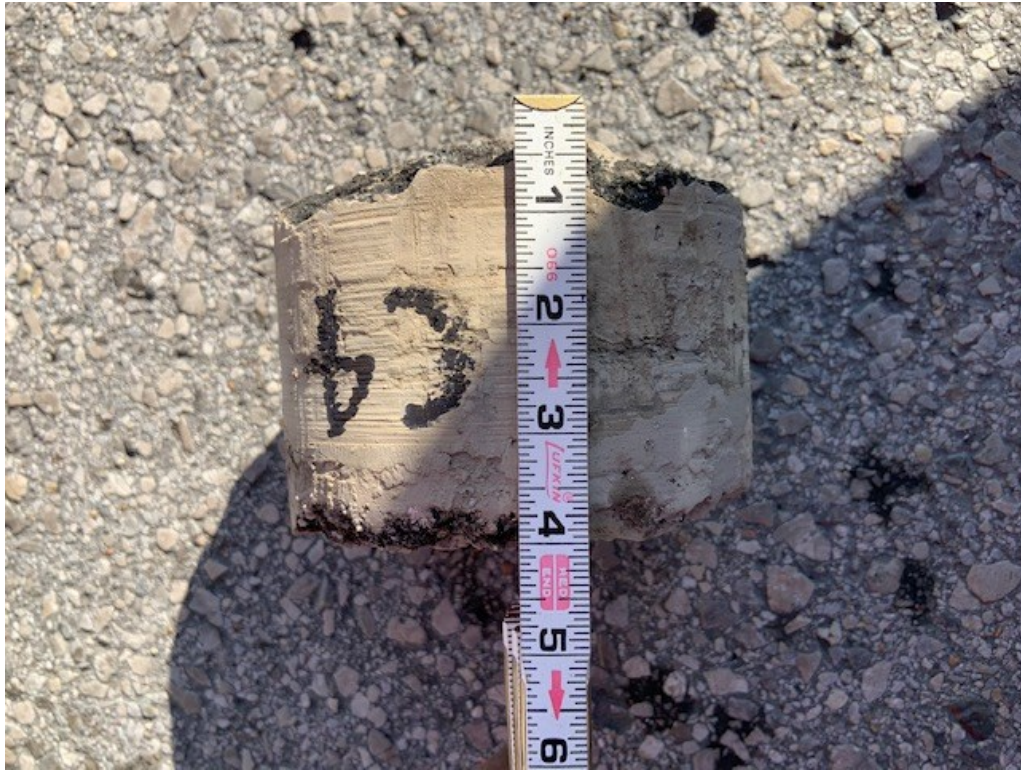
Fig. 9 – C-4: 4 ½” of Asphalt (~1/2” of Sample Left in Hole)
