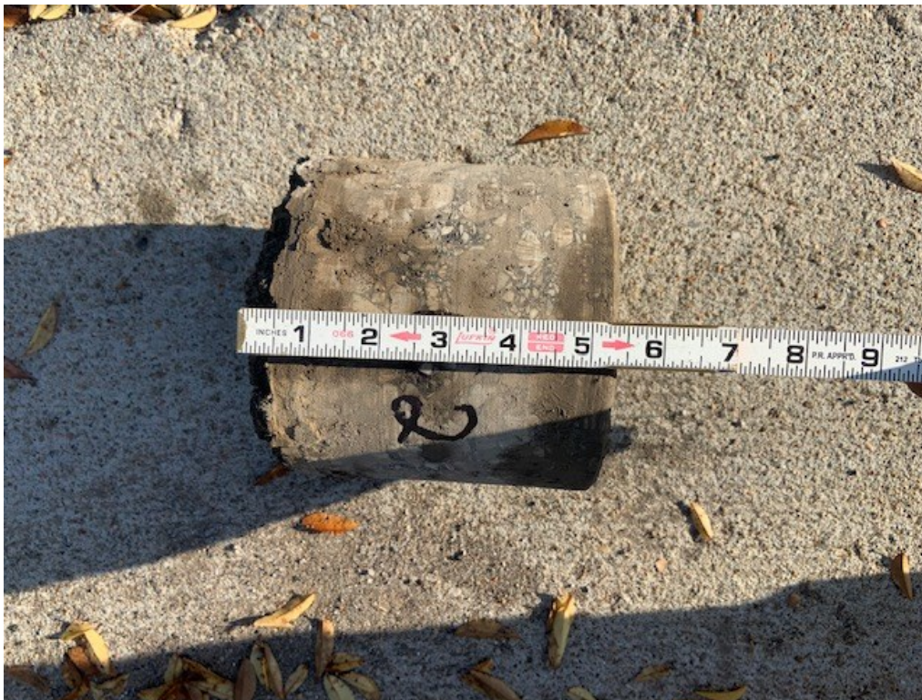
Fig. 4 – C-2: Approximately 5" of Asphalt.
