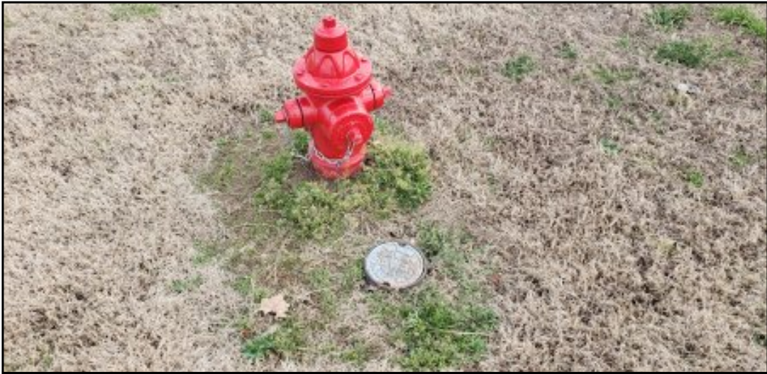
Photo 31: Fire hydrant and water access located on Lot 8.
