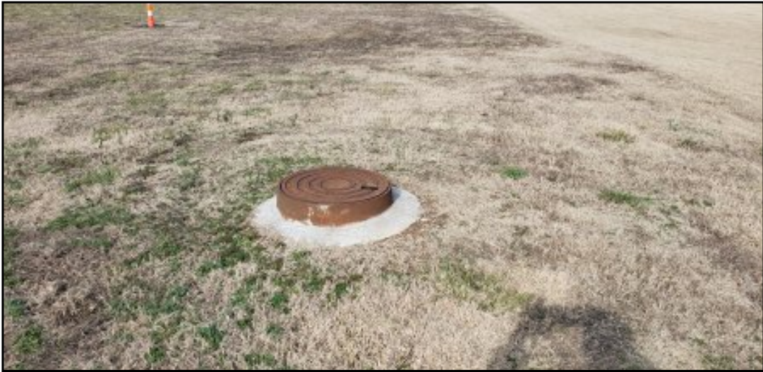
Photo 17: Sanitary sewer access located on Lot 8.
