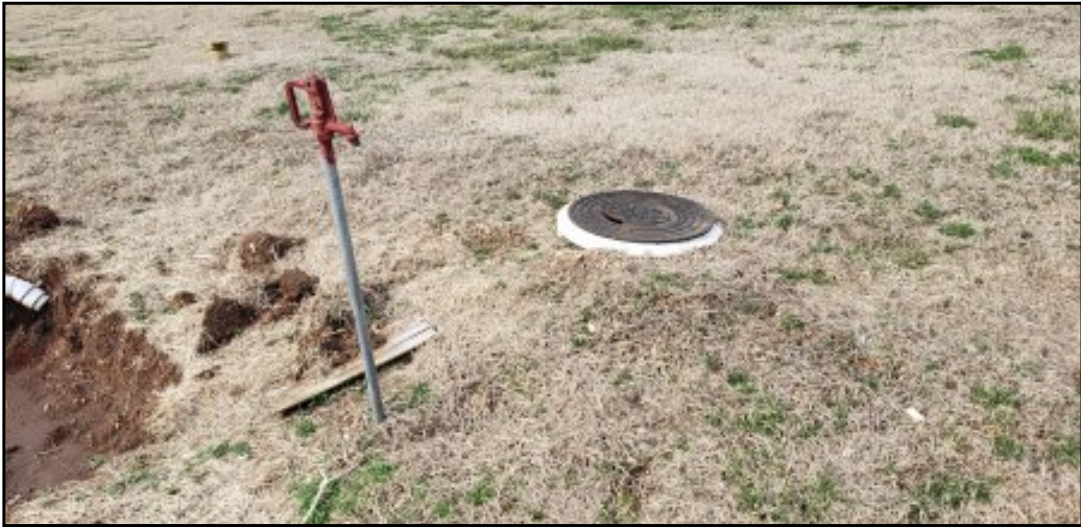
Photo 25: Utility access located on Lot 8 where former project trailer was located.
