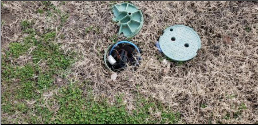
Photo 05: Sprinkler system access located just south of the subject property.
