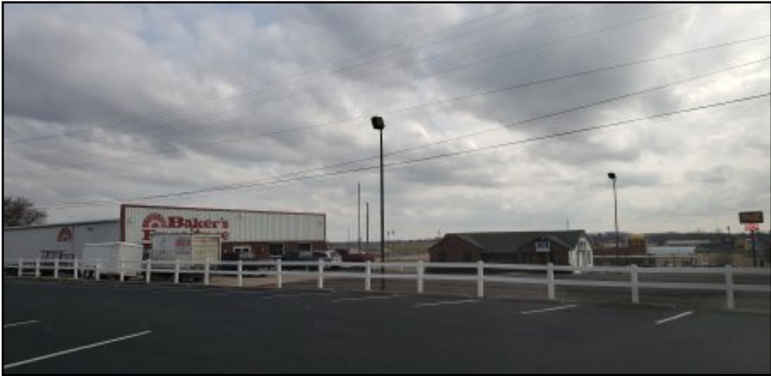
Photo 37: Commercial retail furniture store located just north of Lot 8 and NE of lot 2.
