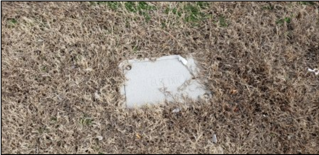
Photo 29: Electric access panel located on Lot 8.
