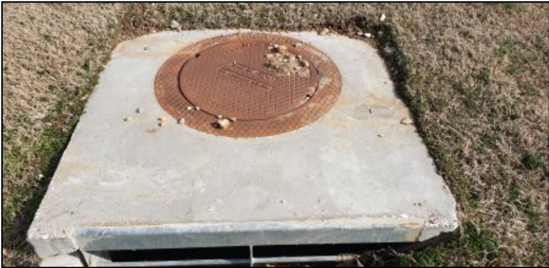
Photo 08: Storm Sewer access located in SE corner of Lot 2.
