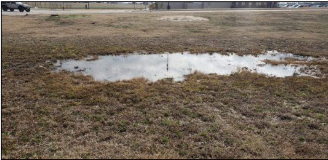
Photo 14: Lot 8 storm water ponding.
