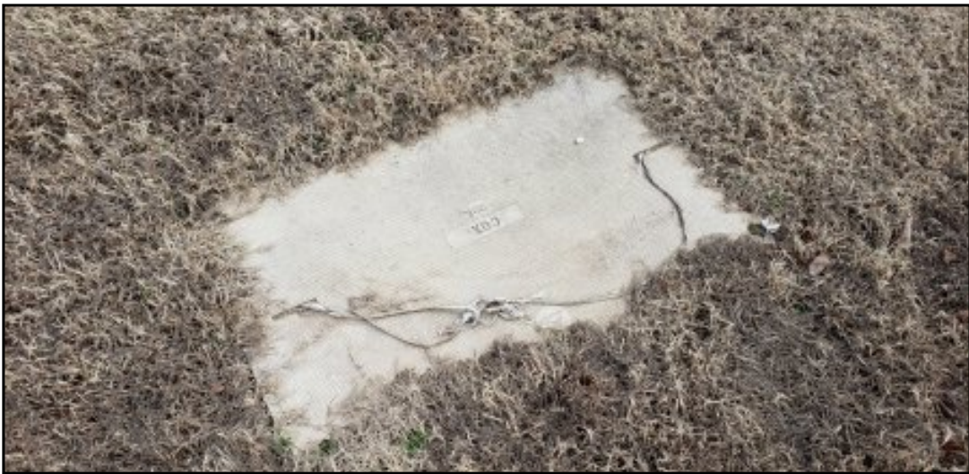
Photo 30: Cox communication access panel on Lot 8.
