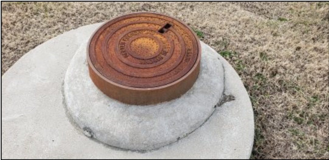
Photo 04: Sanitary Sewer access on Lot 2.
