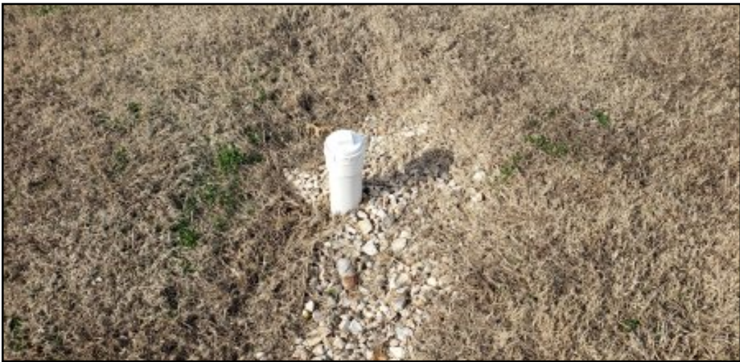
Photo 16: Utility access on Lot 8.
