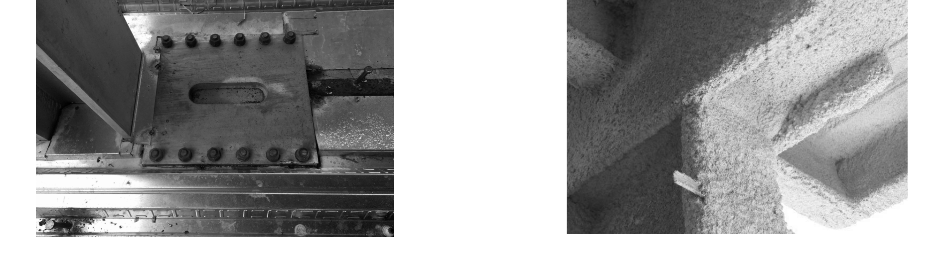
GRAPHIC NO. 9 - TYPICAL GAP CLOSURE AT THE TOP OF THE GAP
