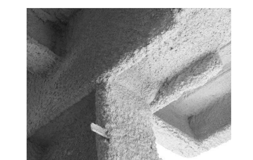
GRAPHIC NO. 10 - FIREPROOFING ACROSS THE BOTTOM OF THE GAP
