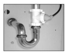
The Drain Line Adapter must be above trap outlet pipe
