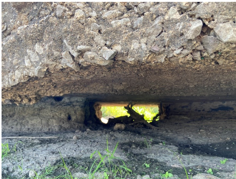
Figure 2: Void underneath the existing concrete weir structure
