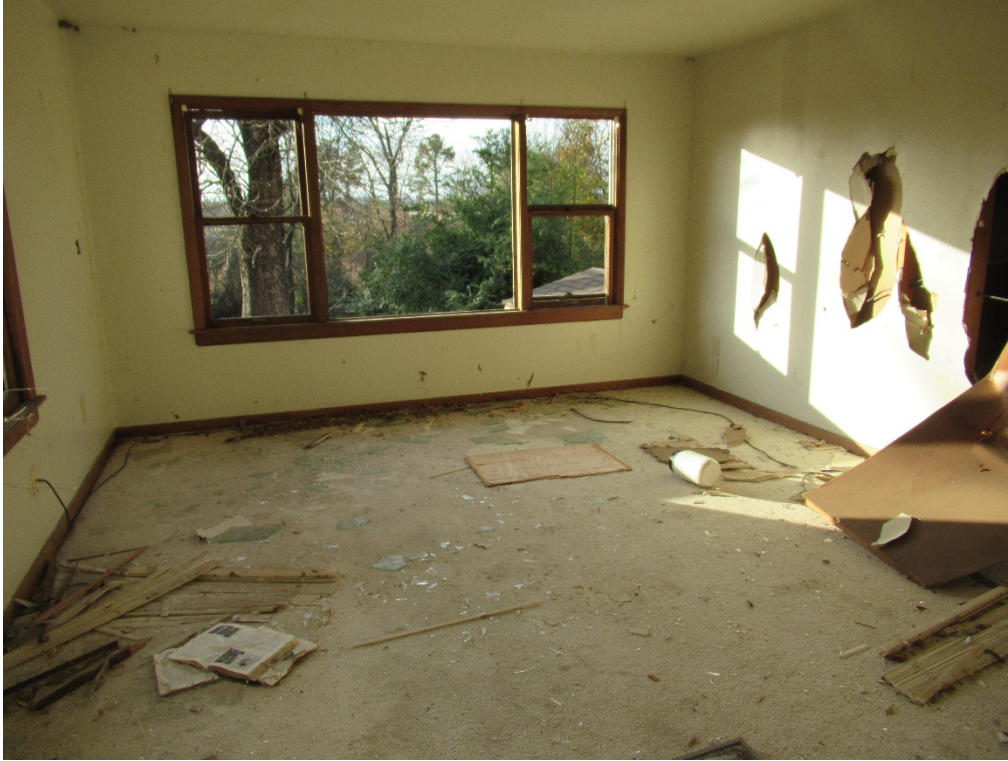
Photograph 1: Wall and Ceiling Texture 3% Chrysotile Asbestos
