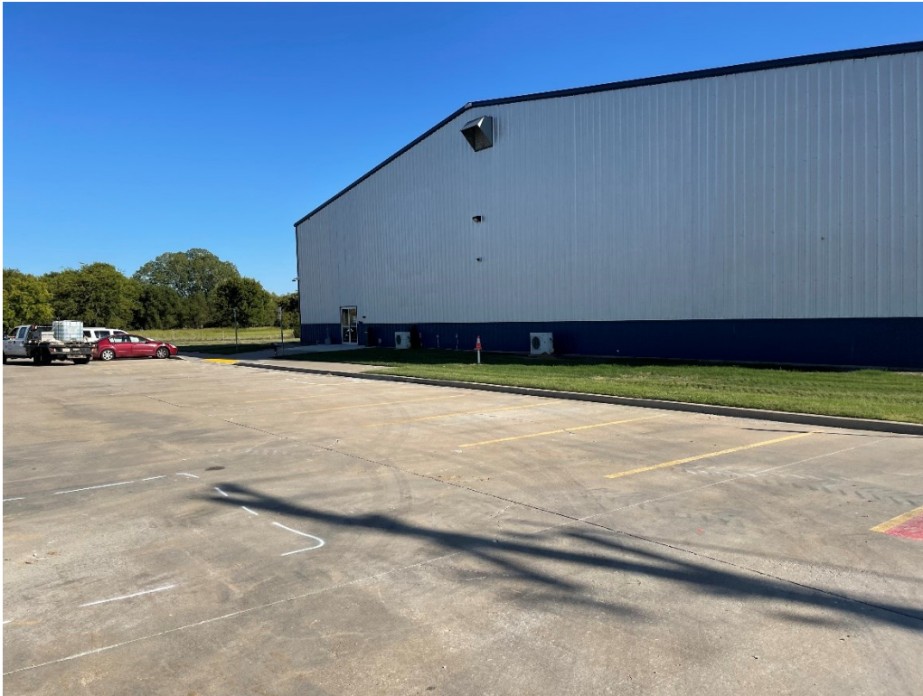
Figure 4: North of the existing building, near boring S-01, looking southeast
