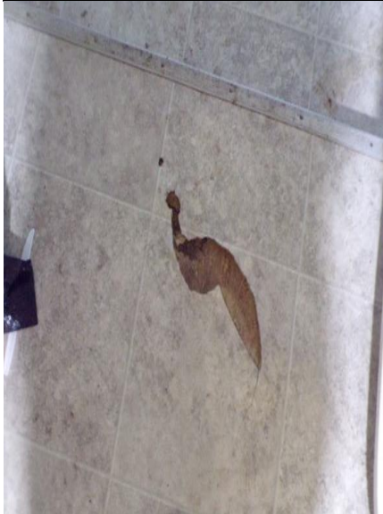
Example of the Cream Sheet Flooring over a wood floor.
