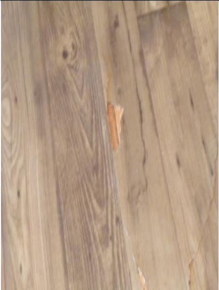
Example of the Brown Sheet Flooring over a wood floor.
