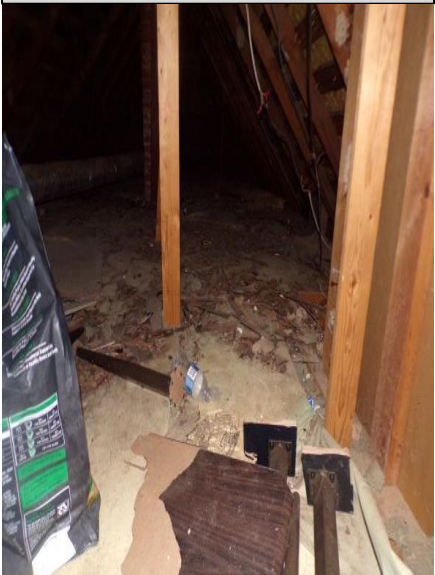
Example of the attic insulation.
